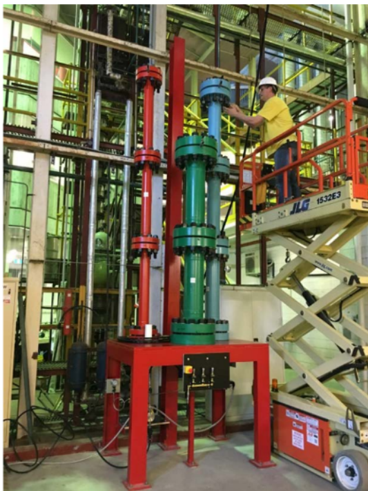
Figure 24: The Well Simulator Facility at the University of Queensland. 4, 6 and 8" pipes (red, blue and green) can be installed and tested up to a maximum pressure of 1000psi. Each pipe is 1m long. Sections of up to 5m height can be installed. Pressure transducers are installed at the flanges and allow pressure monitoring while pumping.
